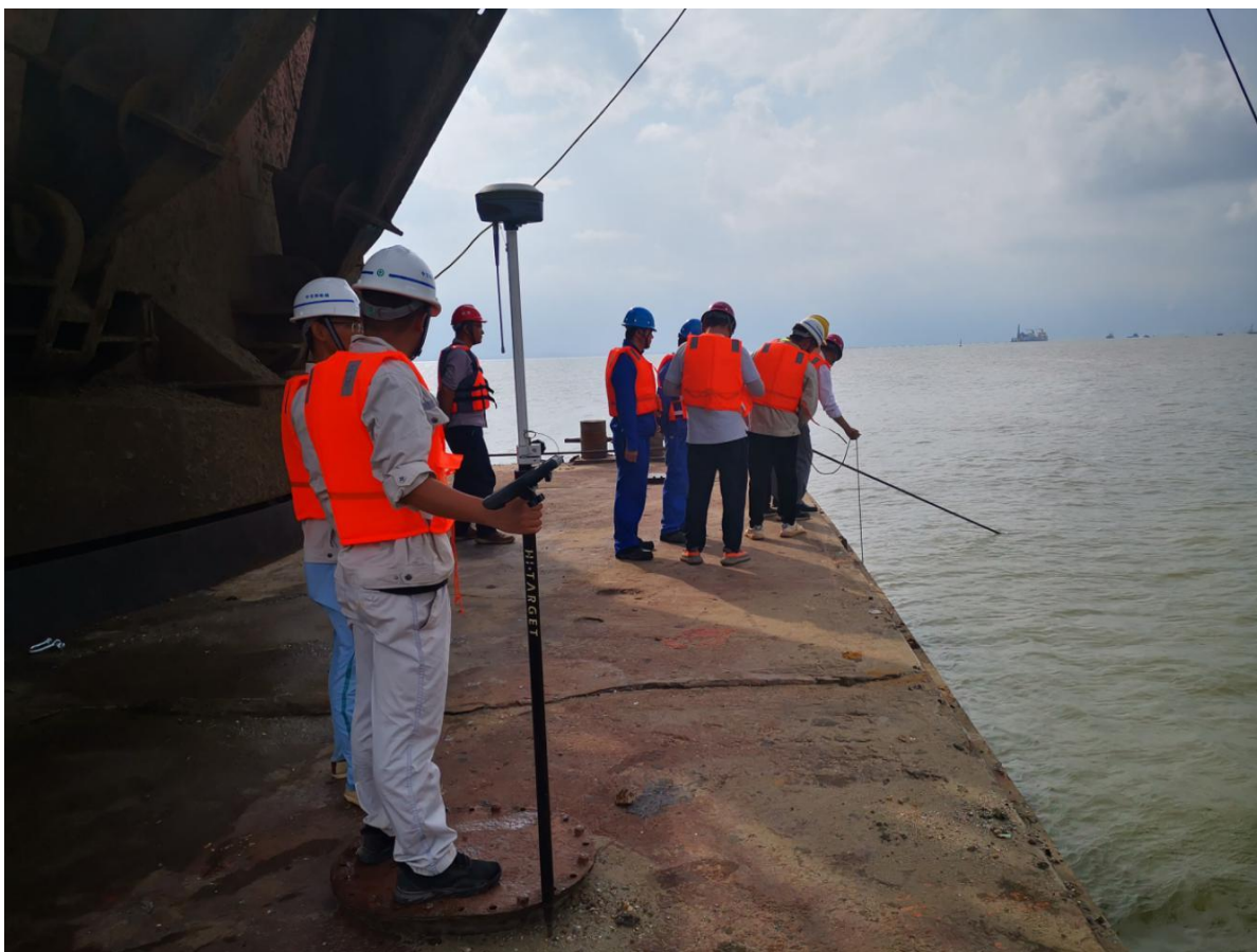
2#码头基槽挖泥验收
